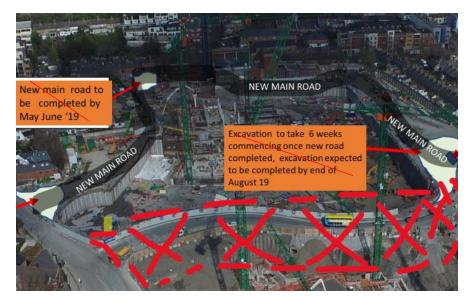
The excavation will take approximately 8 weeks and sees a relatively small amount of earth left for excavation, but it is approximately 50,000 cubic meters a substantial amount of earth involving relays of McGuire lorries back on the move.
